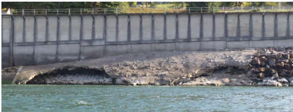
Figure 3 – Photo in 2016 of Area Repaired in 2012
